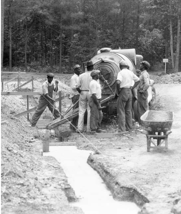
In June 1935, construction of the Museum's Great Hall began. Shipyard workers pour footing; the first library section is at right. From The Mariners' Hidden Histories Collection. The Mariners' Museum and Park INST-EX-267_02
